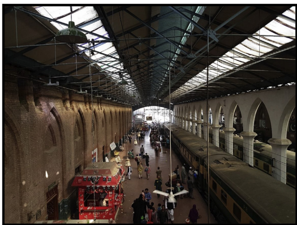
Fig. 12 Gothic Arches in red bricks and white plaster on both sides of Railway Station.
