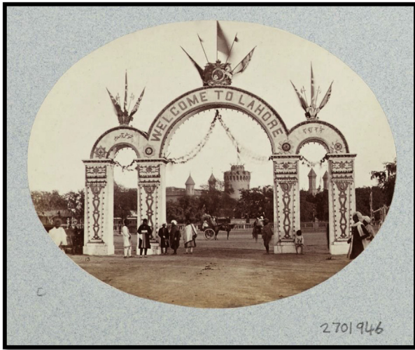
Fig. 5 The archway built near railway station to welcome prince of whales in 1875. Source: Royal collection trust.
